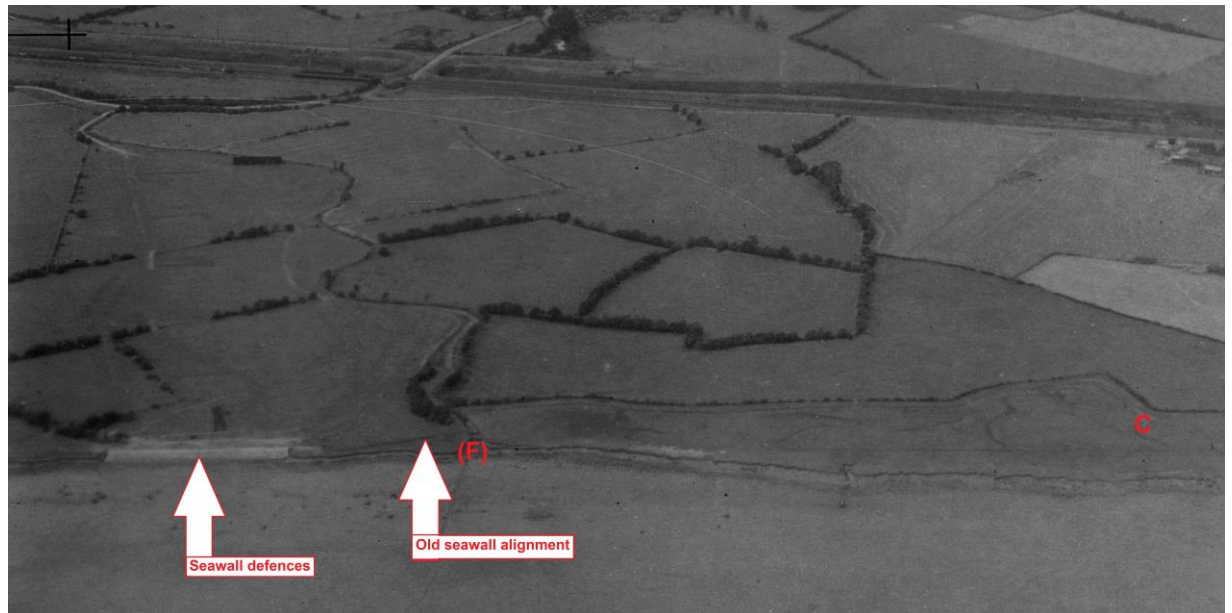
Photograph B: showing 1951 Seawall construction
