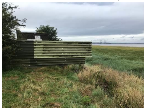
Barrier that westernmost sentry box
